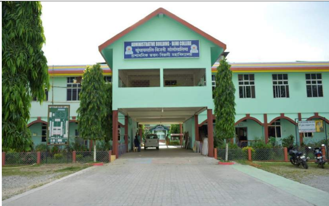
COLLEGE ADMINISTRATIVE BUILDING
